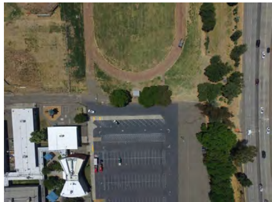
Drone aerial photograph of the LNWI sewer easement at Grande Vista Avenue, looking southbound.
