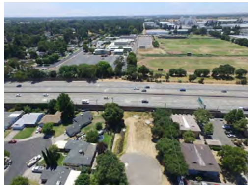
Drone aerial photograph of Westmore Oaks Elementary School and the LNWI sewer easement slightly north of US 50, looking southbound. Source: Drake Haglan & Associates, 2017
